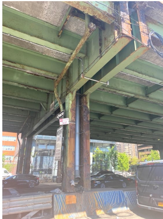
Figure 20. Shows the rusting of the pillar from runoff. The bridge has FDR Drive and the road underneath is FDR Service Road.
