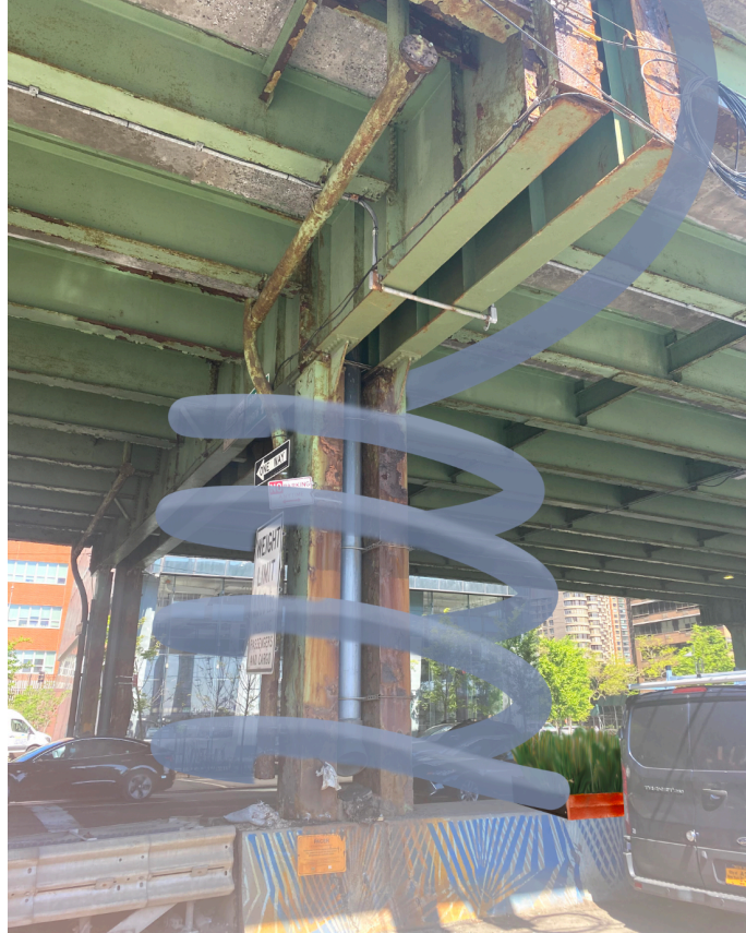
Figure 23. Rain gutter spiraling down a pillar leading to a raingarden.
